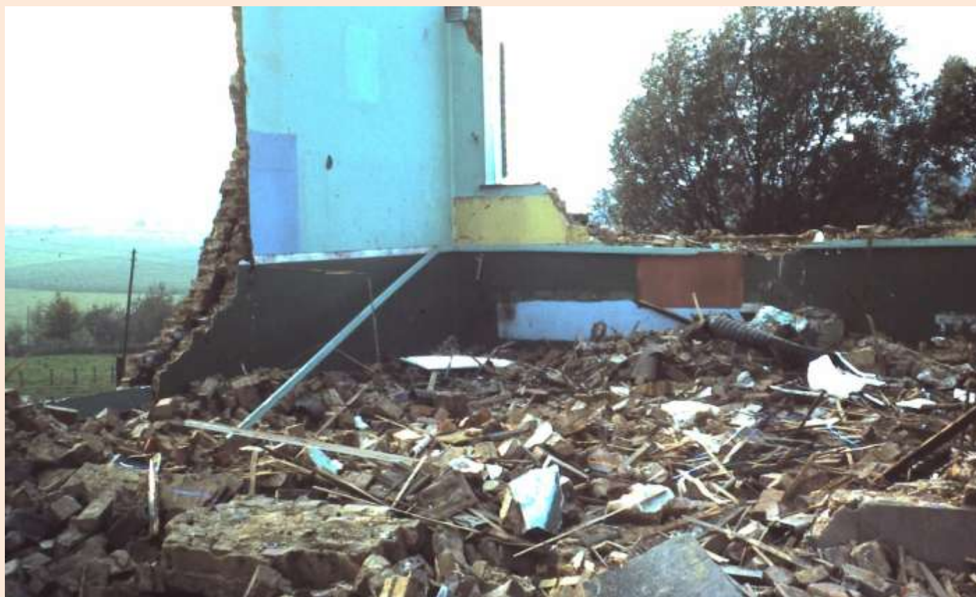
School in puin
