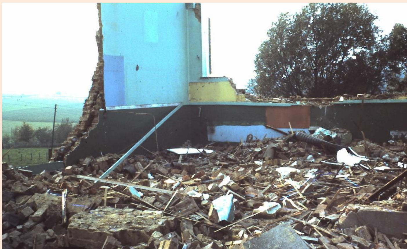
School in puin
