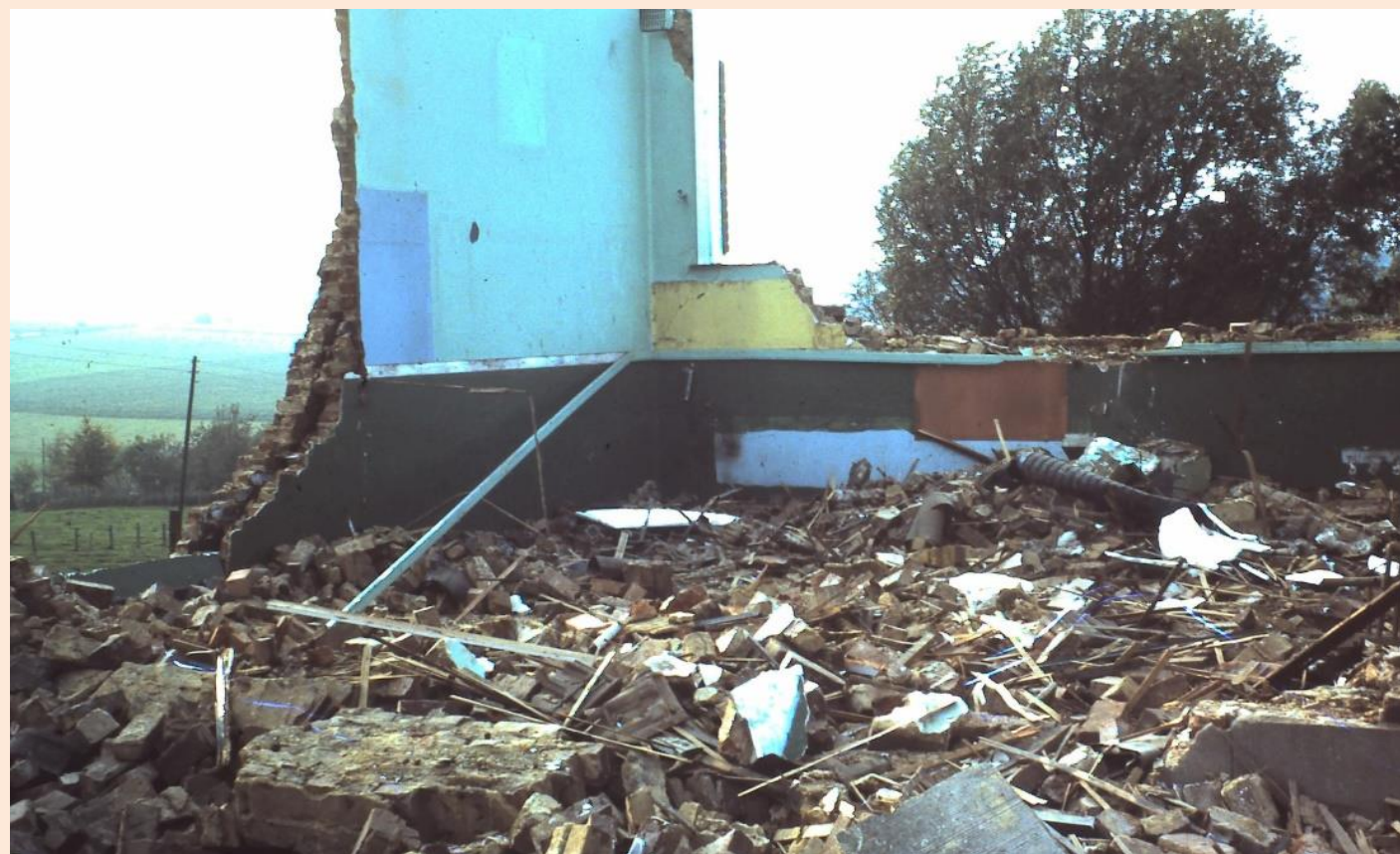
School in puin
